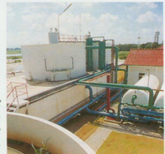
CLEARWELL UNDER THE CLARIFIER AT SIAM CEMENT INDUSTRIAL ESTATE'S WTP
