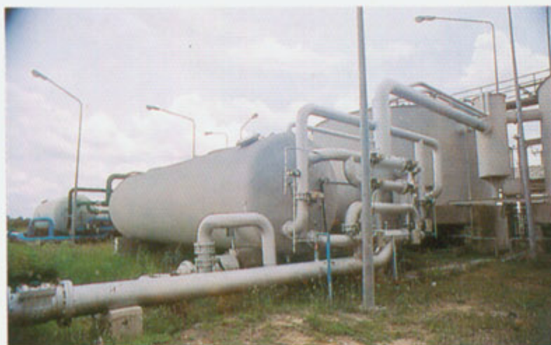
PRESSURE SAND FILTERS WELLGROW INDUSTRIAL ESTATE
