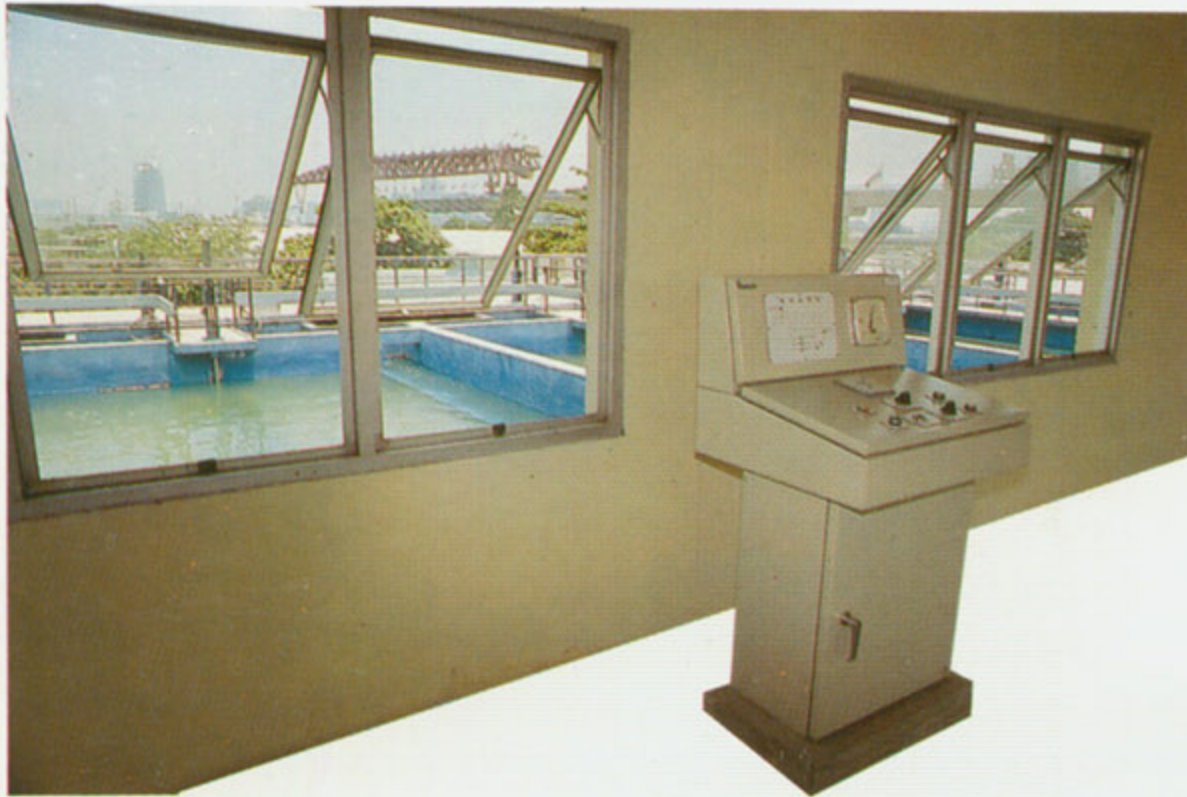
AUTOMATIC CONTROLLER FOR THE FILTERS SAMSEN WATER TREATMENT PLANT, BANGKOK, MWA
