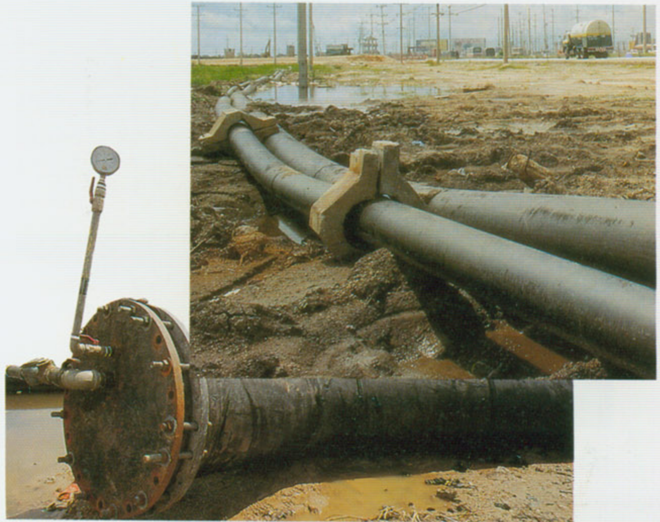
HDPE PIPING FOR WATER TRANSMISSION NETWORK, BANGPAKONG, CHACHOENGSAO
